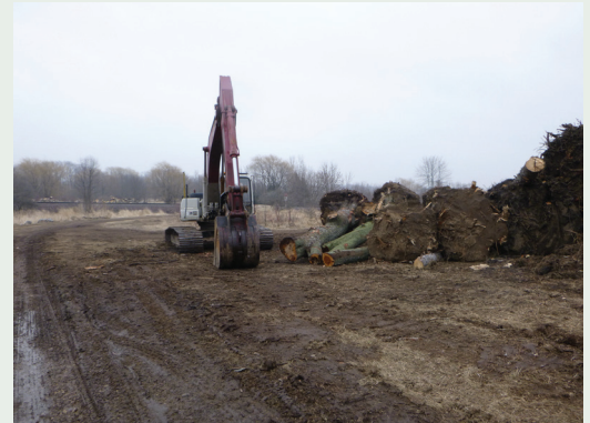
The project will incorporate salvaged large woody debris for bank stabilization and habitat structure
