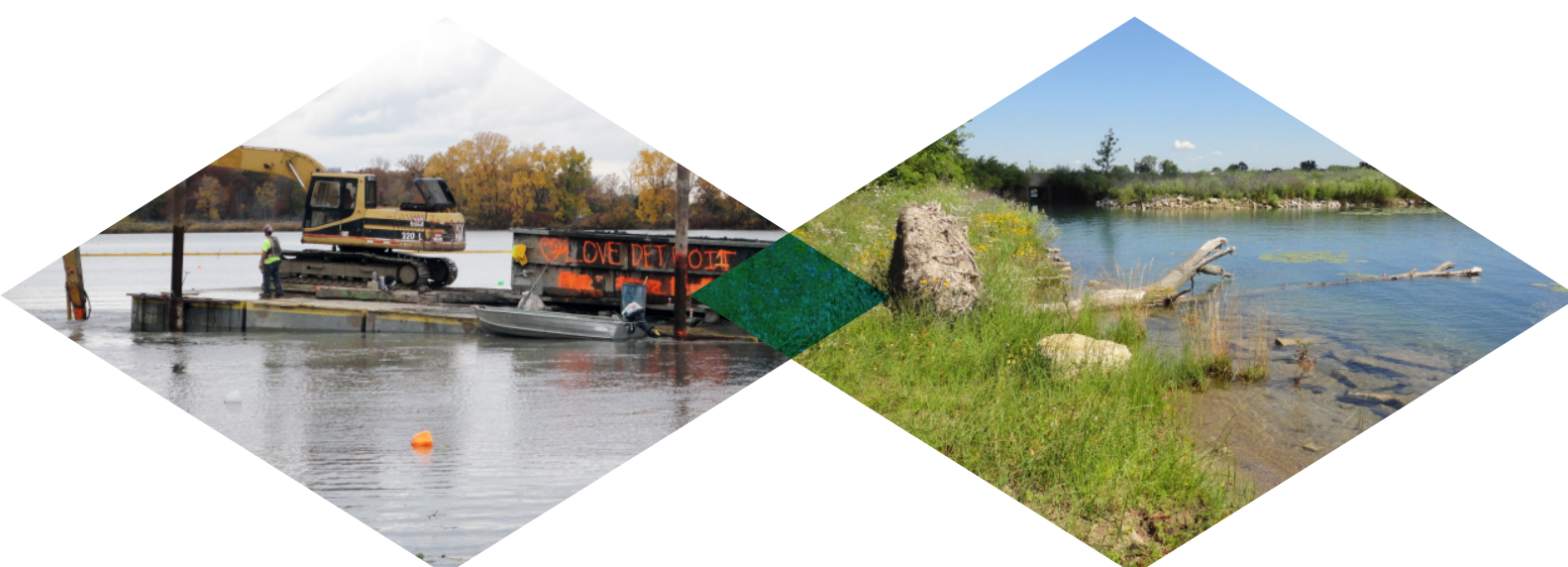
Friends of the Detroit River has leveraged grants from the HOW Grant Program into several restoration projects in the Detroit River. The photo on the left depicts a project on the west end of Belle Isle: an excavator on a barge moves sediment from one location to another in the Blue Heron Lagoon. By changing the depth of the water column, a variety of habitats are being created. The photo on the right shows native species planted around Blue Heron Lagoon, both in and around the water. Native wildlife will be able to thrive thanks to the work of student volunteers. Photos courtesy of Friends of the Detroit River.
