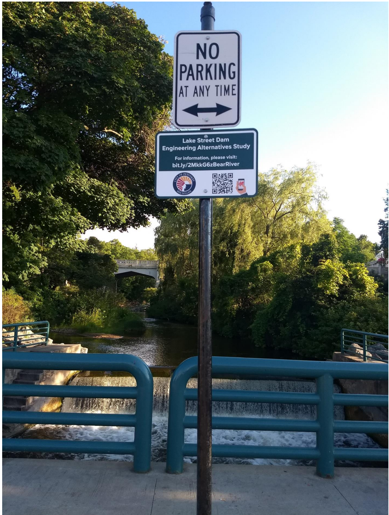
Figure 4: Signage posted at dam
