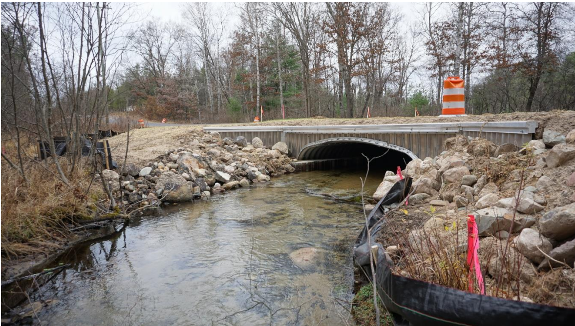
Newly installed structure outlet (Blood Creek/72 nd Street)
