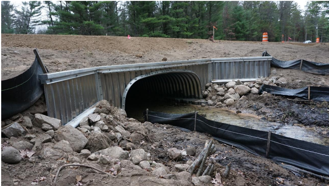
Newly installed structure outlet (Blood Creek/Broadway Avenue)
