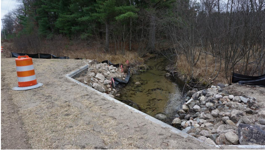
Newly installed structure inlet (Blood Creek/72 nd Street)
