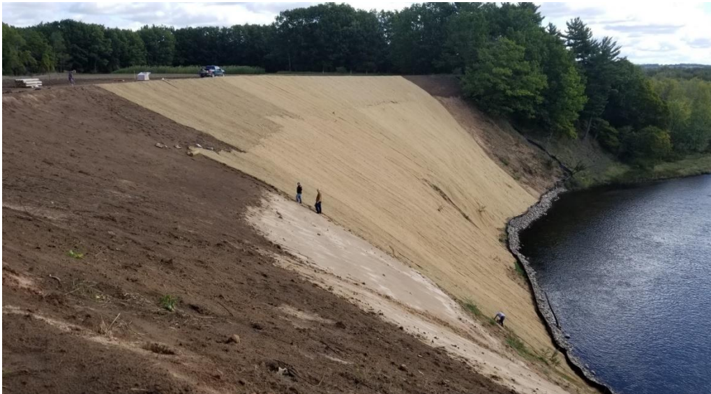
Chinnery Rollway slope stabilization
