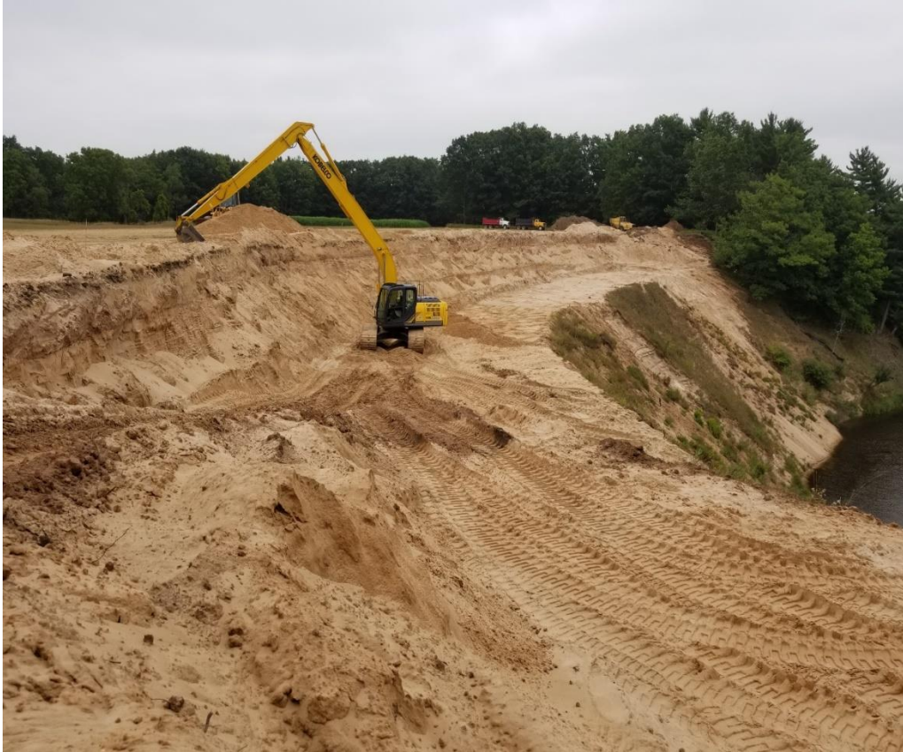
Chinnery Rollway work progressing
