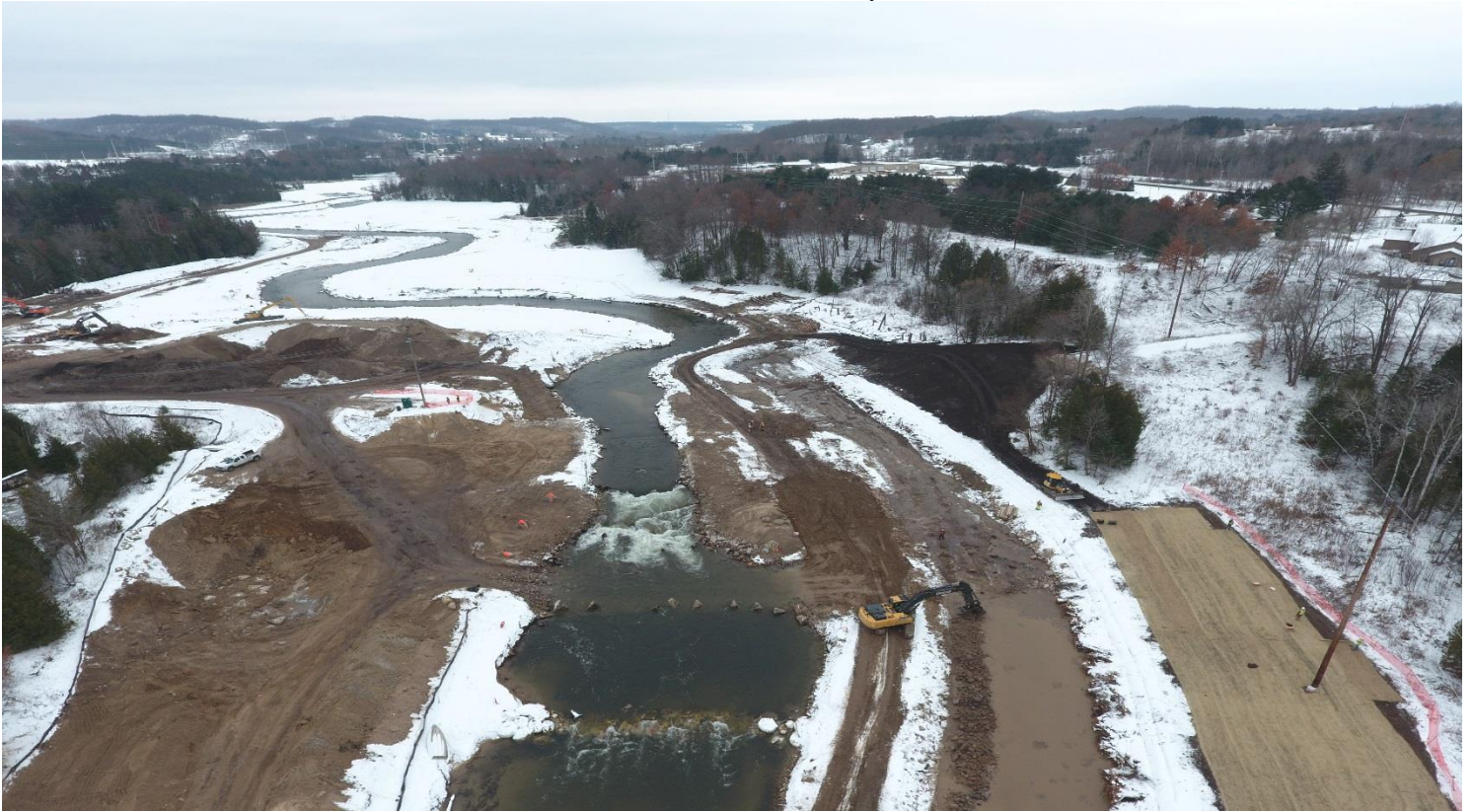
Aerial of Sabin Dam December 11, 2018. Photo by GTB Natural Resources.
