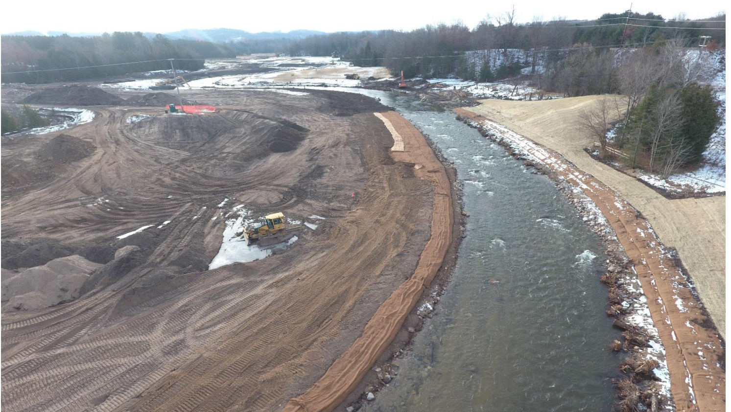
Aerial of Sabin Dam December 19, 2018. Photo by GTB Natural Resources.
