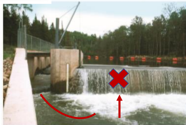
Fishway at Brule River sea lamprey barrier, Wisconsin.
