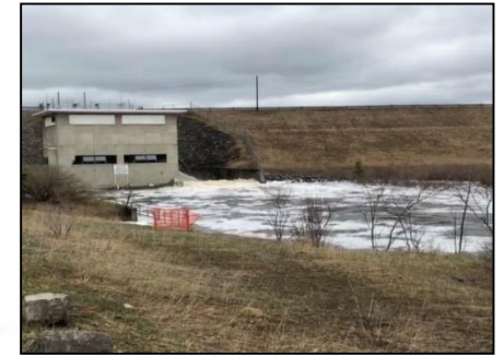
Kleber Dam on Upper Black River
