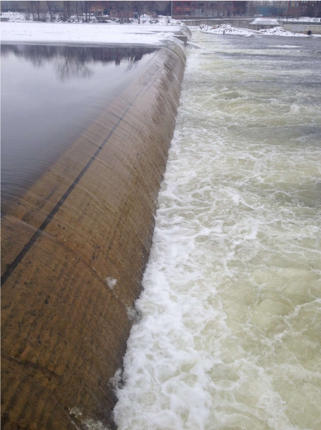
Figure 1. Existing 6 th Street Dam
