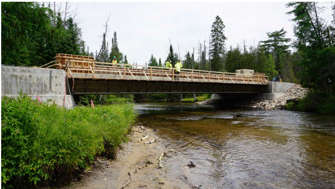
Getting ready to pour the end sections & side walls of the bridge rails.
