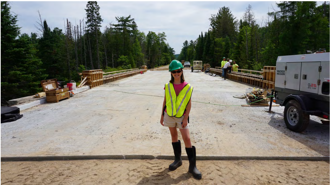
Bridge deck looks awesome & accommodates two 6' wide shoulders & two 11' wide vehicle lanes for a total width of 34' versus the former 25' width.
