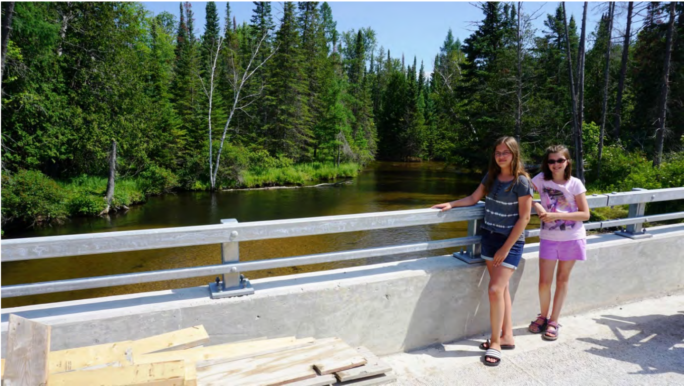
After - Bridge rails are 54" high & have parapet tubing; they are safe for both pedestrians and vehicles.
