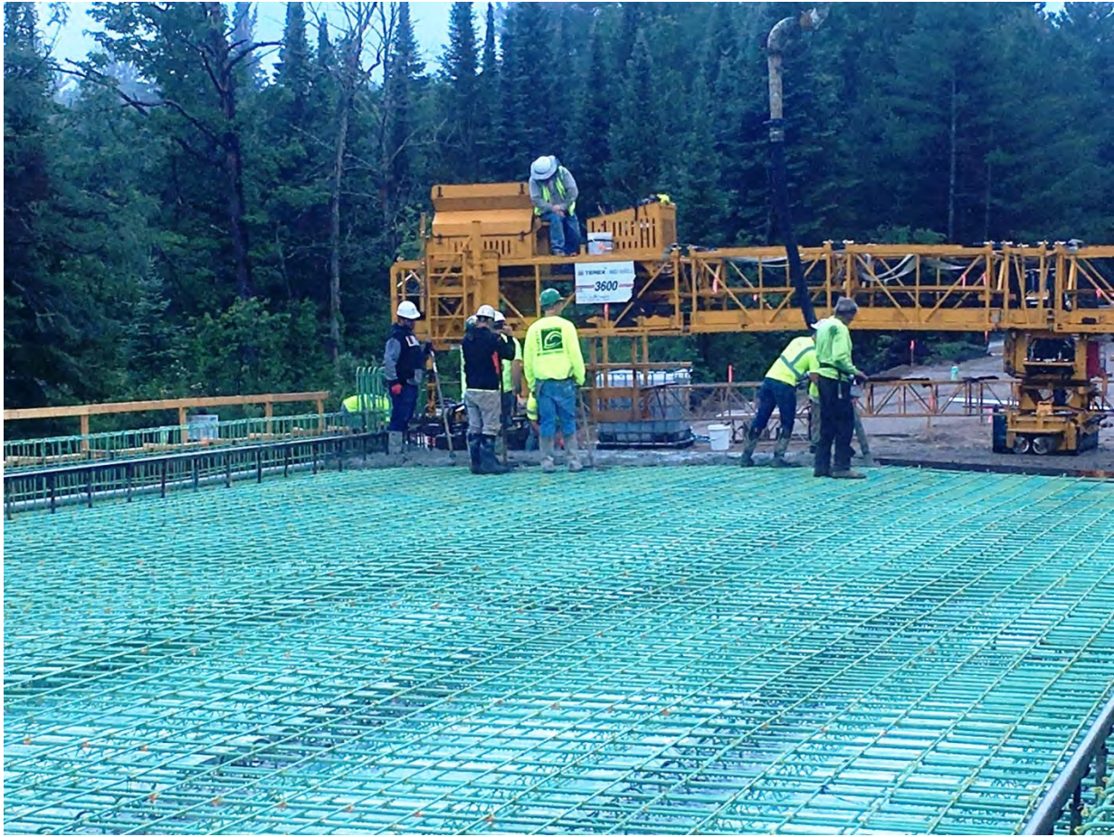
Bridge deck looks awesome & accommodates two 6' wide shoulders & two 11' wide vehicle lanes for a total width of 34' versus the former 25' width.
