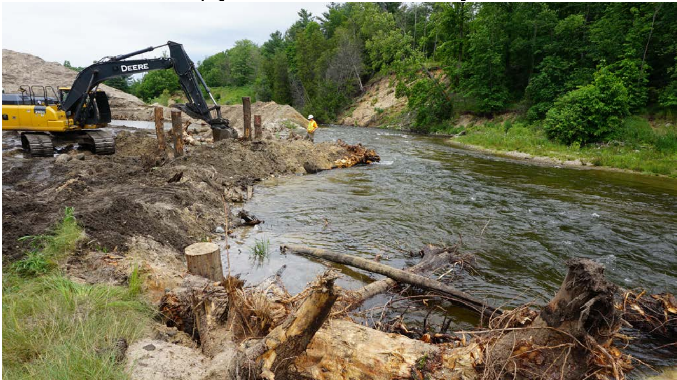
June 2017 – Burying rootwads in streambanks & anchoring with more wood.
