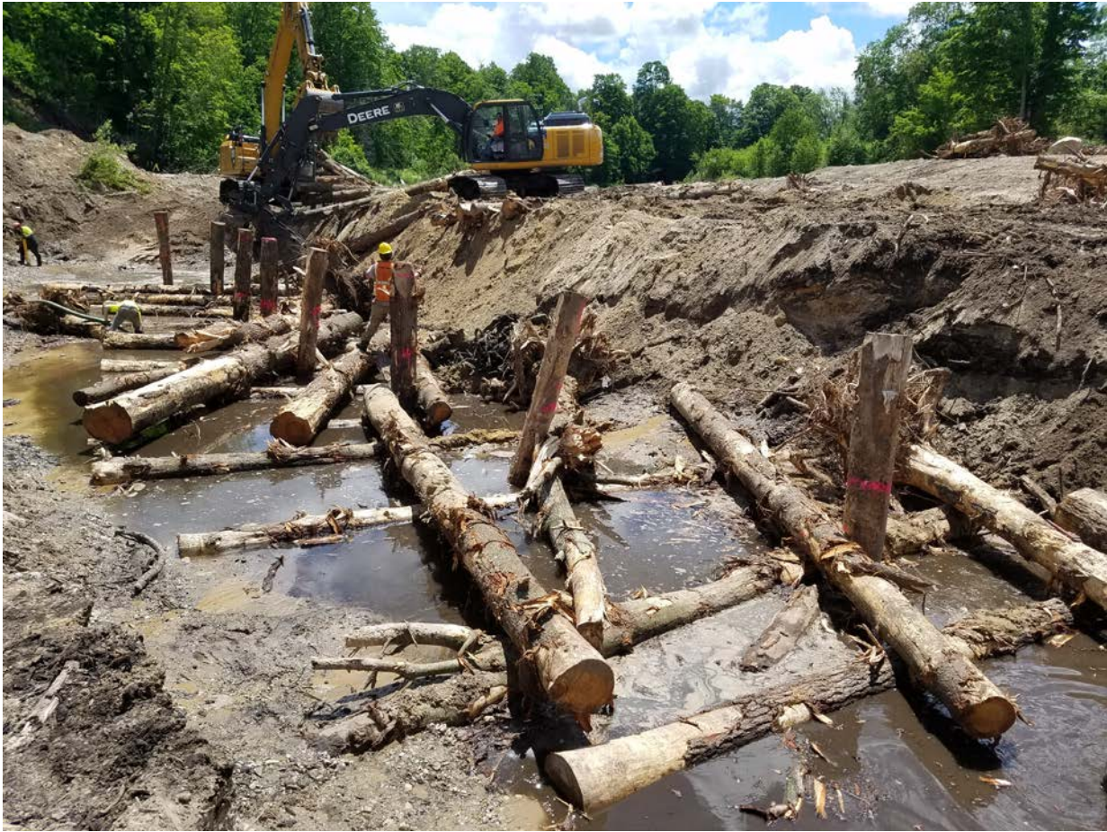
June 2017 – Burying rootwads in streambanks & anchoring with more wood.
