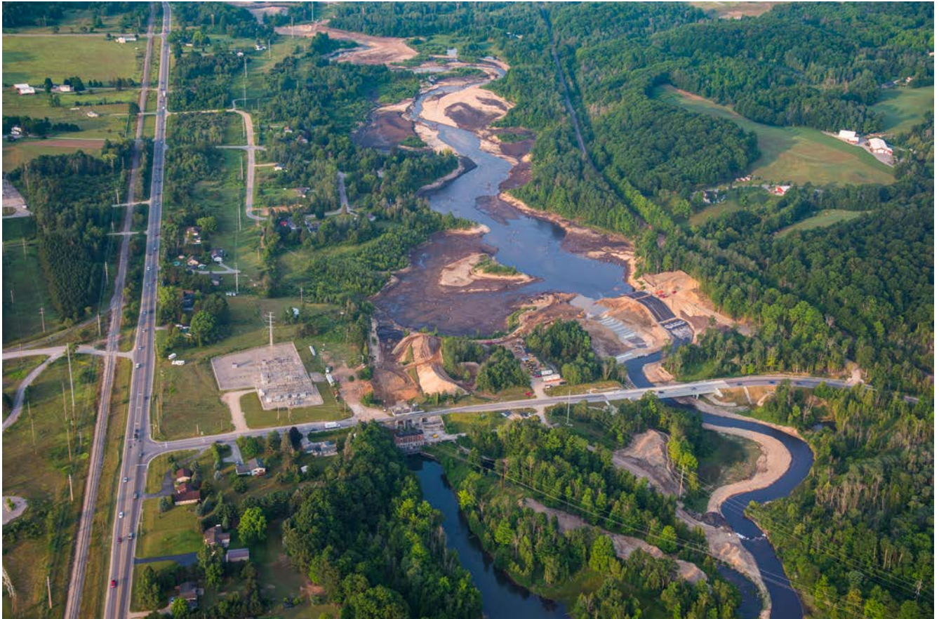
July 2017 – Boardman pond being drawn down with water flowing through siphons & not through the powerhouse.
