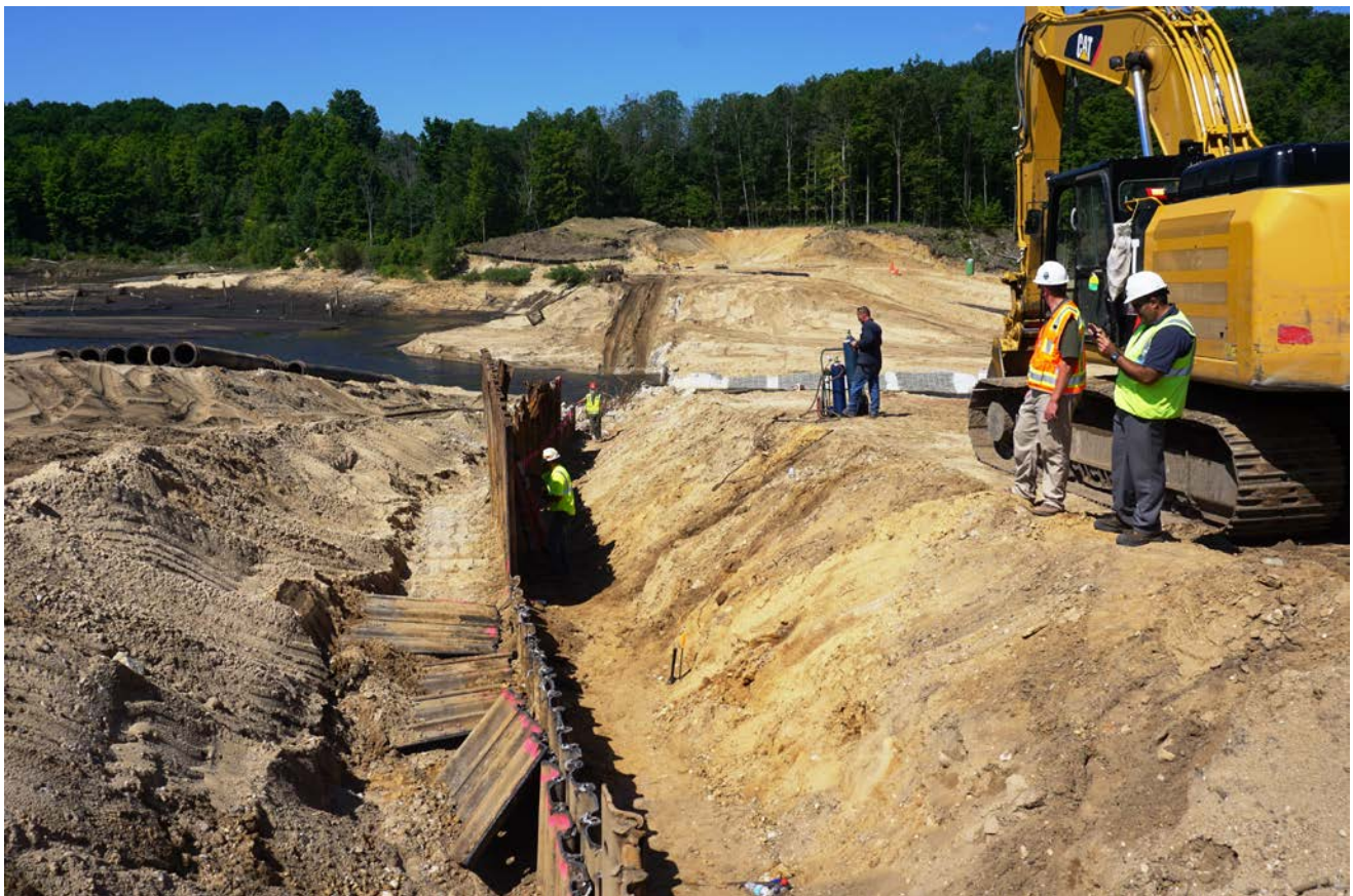
July 2017 - Cutting apart the sheet pile that was underneath part of the concrete wall in the dam embankment.
