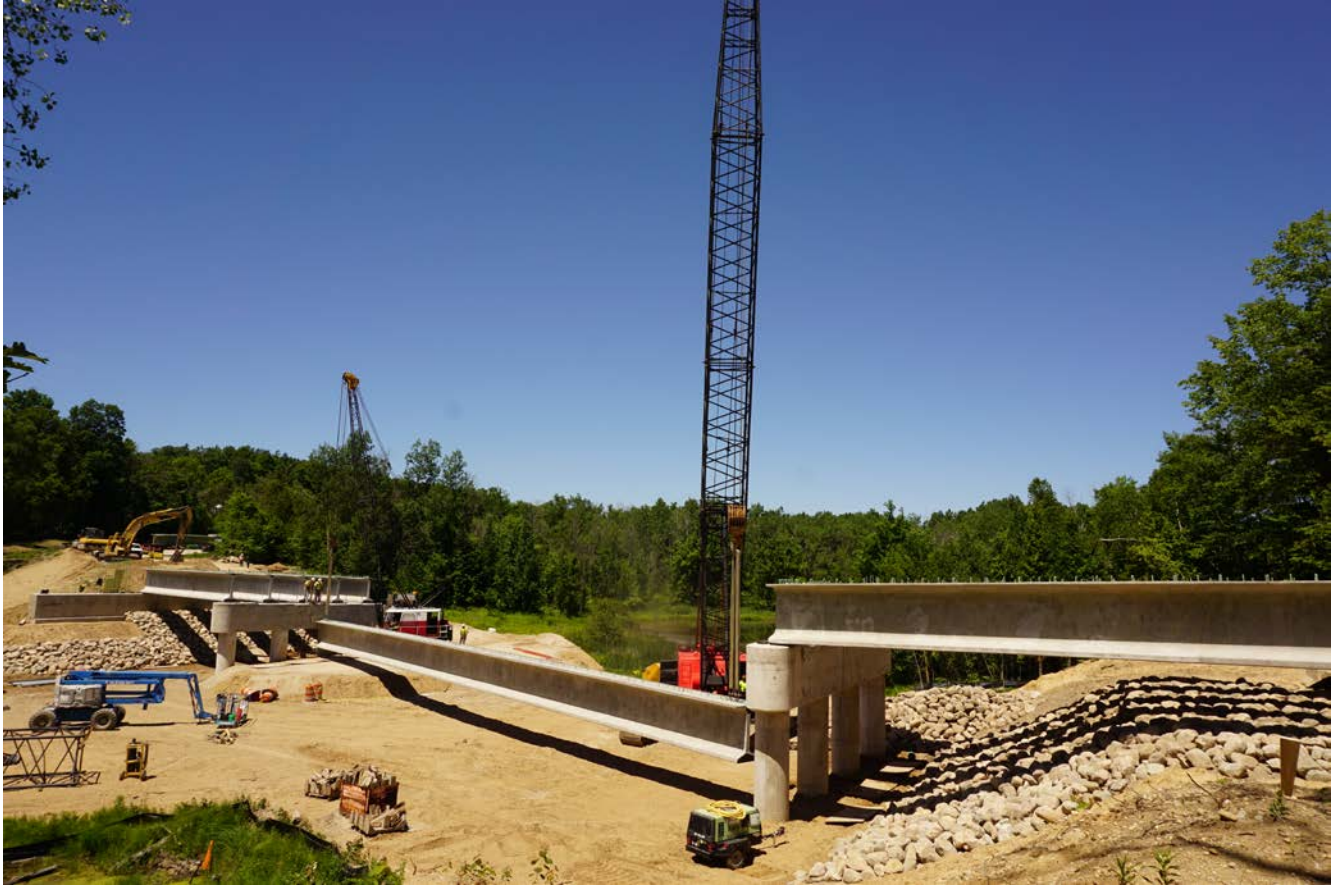
June 2016 - Cass Road Bridge project underway with 135' center beams being set
