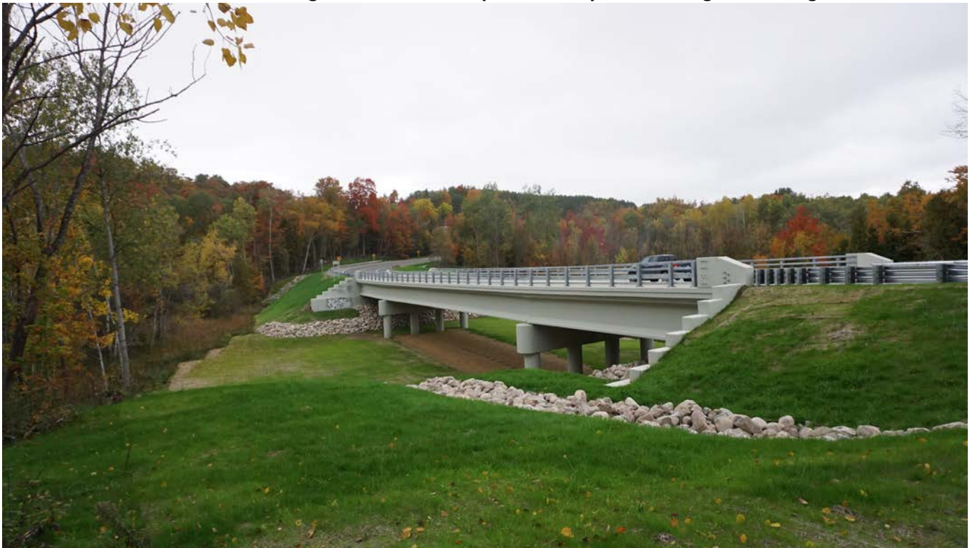
October 2016 – Cass Road Bridge construction complete & ready for returning river to original location
