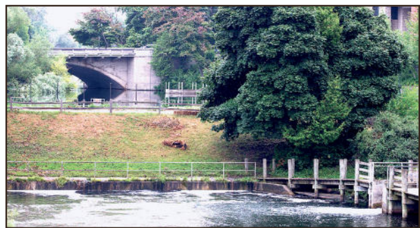
Record-Eagle file photo/Tessa Lighty The Union Street Dam in Traverse City was built in 1867 to power a flour mill. It is planned to be the one dam left on the Boardman River following completion of The Boardman River Dams Ecosystem Restoration Project. It will be modified, but still maintain water levels on Boardman Lake and prevent invasive sea lamprey from getting upstream.
