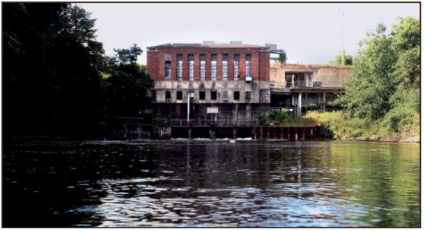
Record-Eagle file photo/Jan-Michael Stump The Boardman Dam was built in 1894 to supply hydropower to the region. It was decommissioned by Traverse City Light & Power in 2005 and now holds water in Keystone Pond in Garfield Township. The Michigan Department of Environmental Quality instructed its owner, Grand Traverse County, to repair or remove it. The Boardman Dam is next in line for removal, slated to start in 2017.
