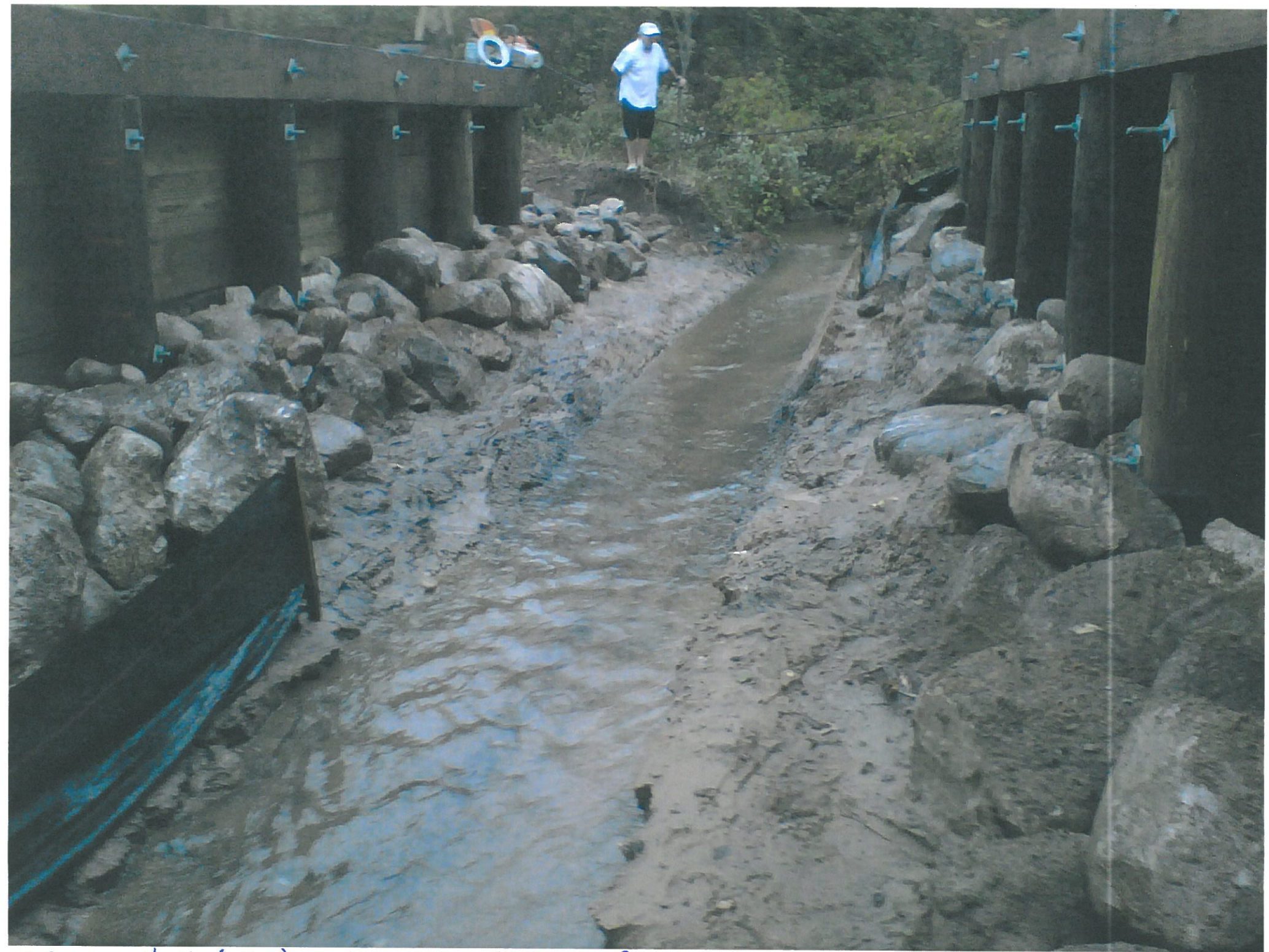
10.3.12 North (inlet) section removed: Creek flowing clean, clear
