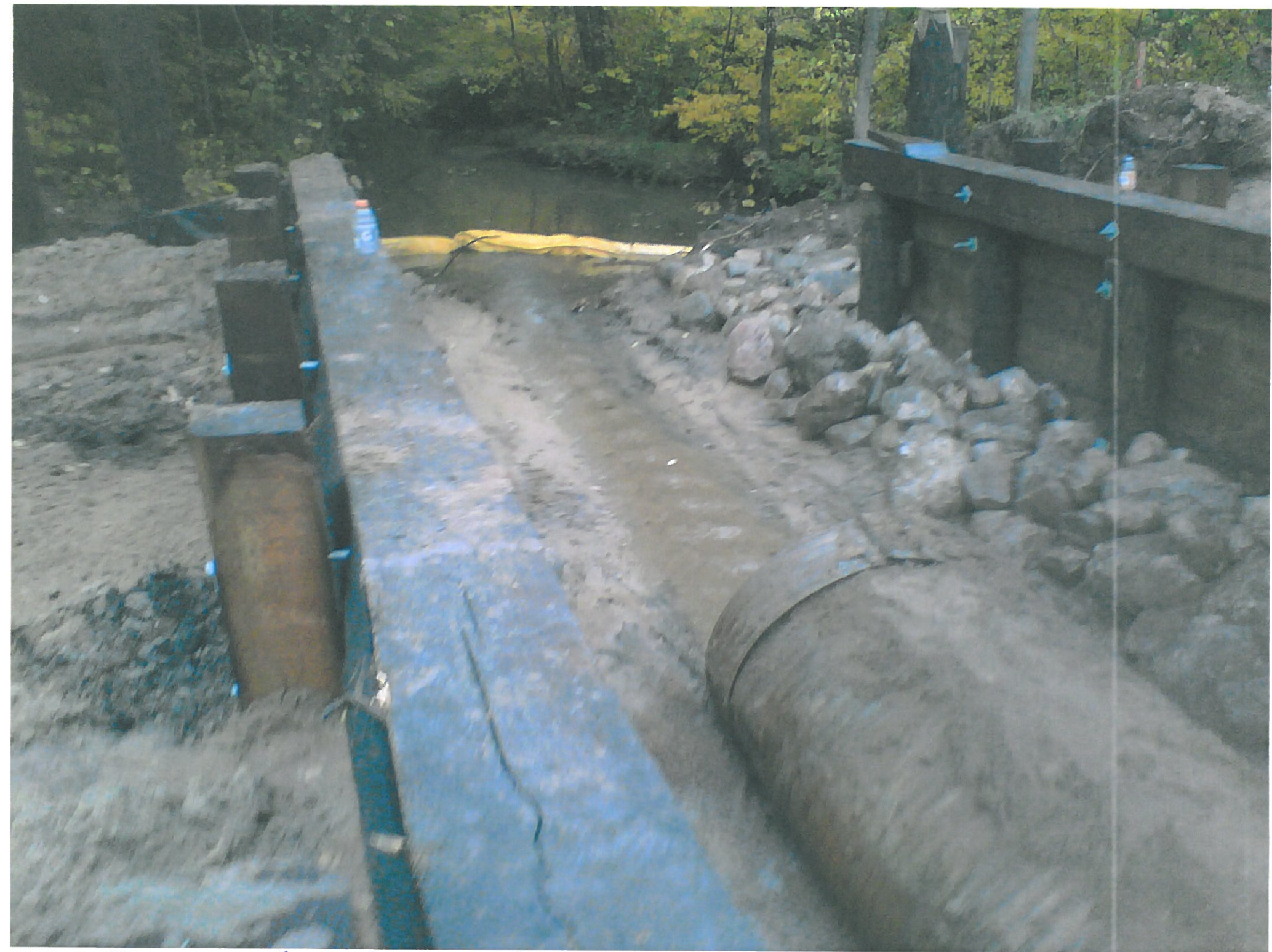
10-3-12 Downstream (outlet) section of culvert removed
