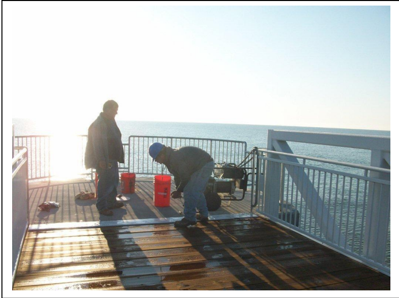
Finishing work pier endcap
