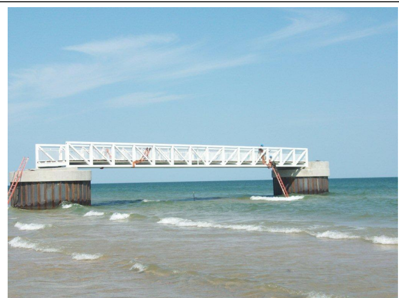
Installed 100' section of pedestrian bridge
