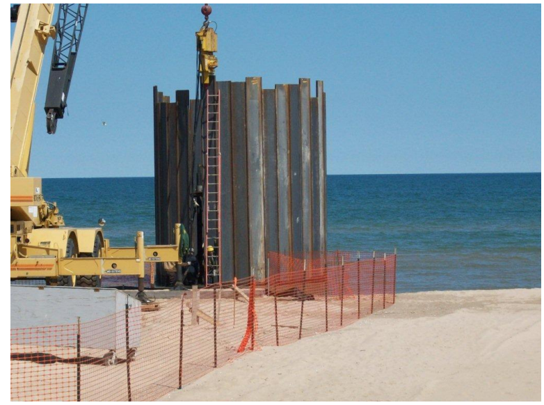
First of three caissons being installed
