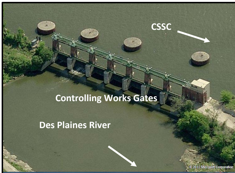
Exhibit 4. Lockport Controlling Works
